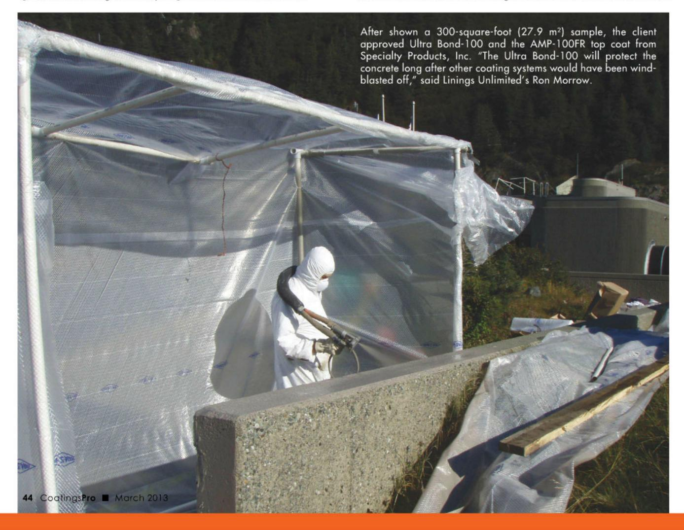
RIGHT • Once prepped, the Linings Unlimited's crew applied the polyurea coating system at a 100-160-mil (2,540-4,064-micron) thickness using a Graco H20/35 Pro. All crew members wore safety goggles, respirators or particle masks, and Tyvek suits.
